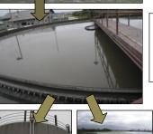
Clarifier: removes organic material to be sent to the digesters for further processing
