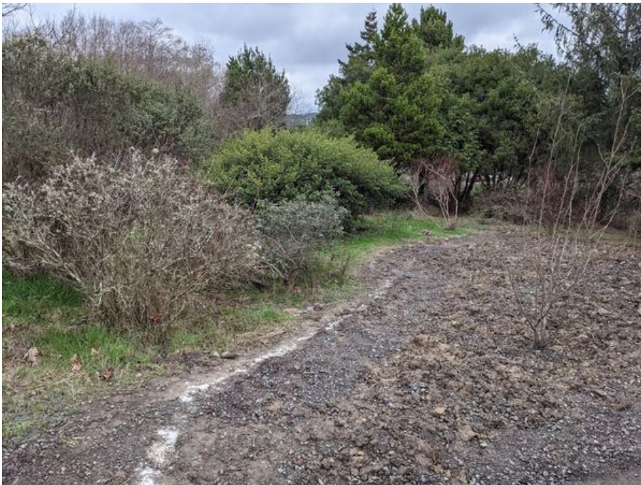
Phase I cleared ground. Photo by Lynn Jones.
