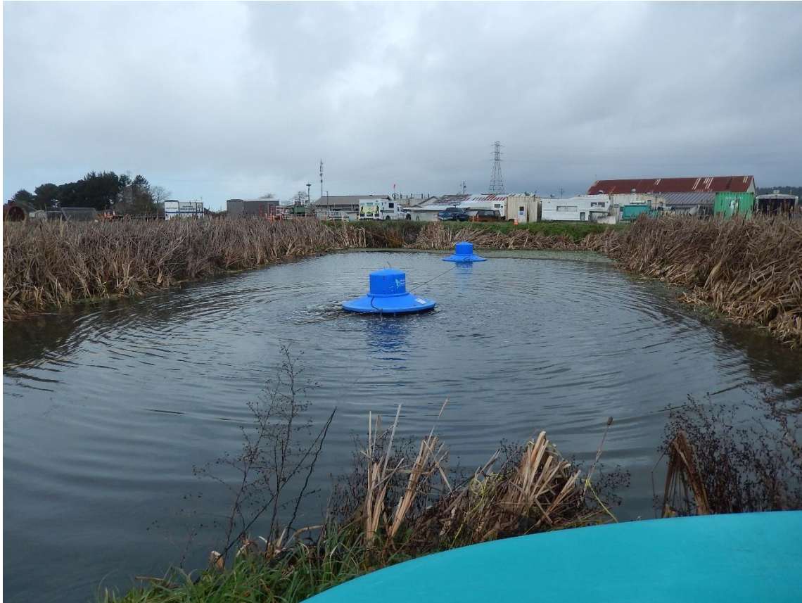
Figure 12.4 Blue Frog circulators helping to reduce the load of organic sludge in Treatment Wetland 3. Photo by Sharon Levy.
