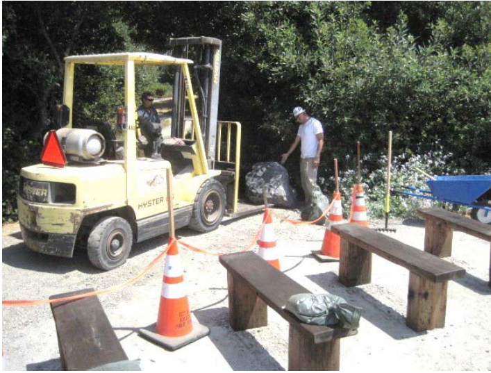
Installing the amphitheater benches. Photo by George Ziminsky.
