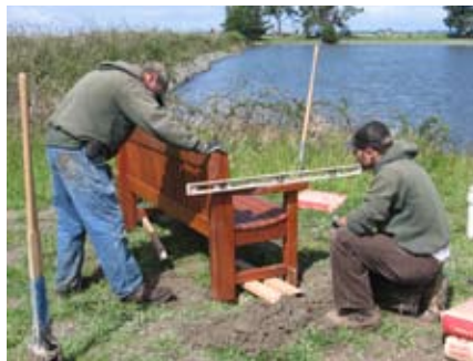
Installing replacement bench at Klopp Lake. Photo by George Ziminsky.
