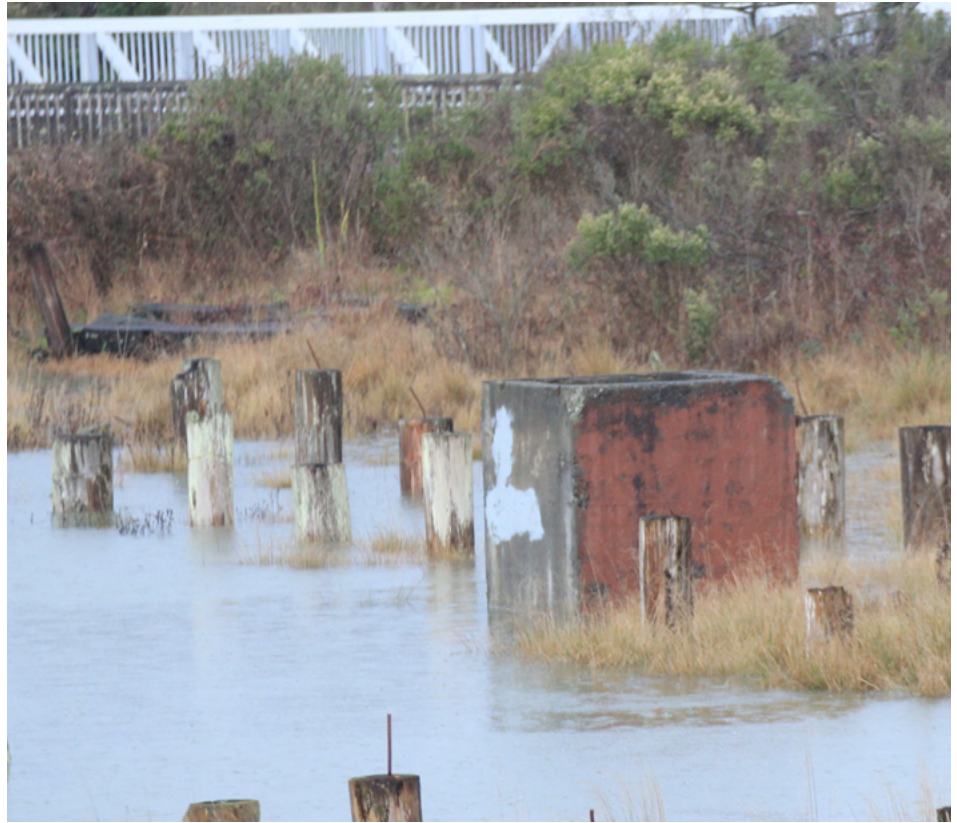
The King Tides filled up Butcher Slough, with the water reaching the concrete structures south of the Interpretive Center. Photo by George Ziminsky.
